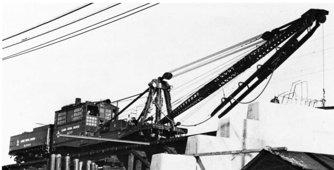
IC X17 STEAM PILE DRIVER. PHOTO BY WILLIAM A. RAIA. Shown during bridge rebuilding at Riverdale, IL in November, 1970. Retired from roster in 1990.
