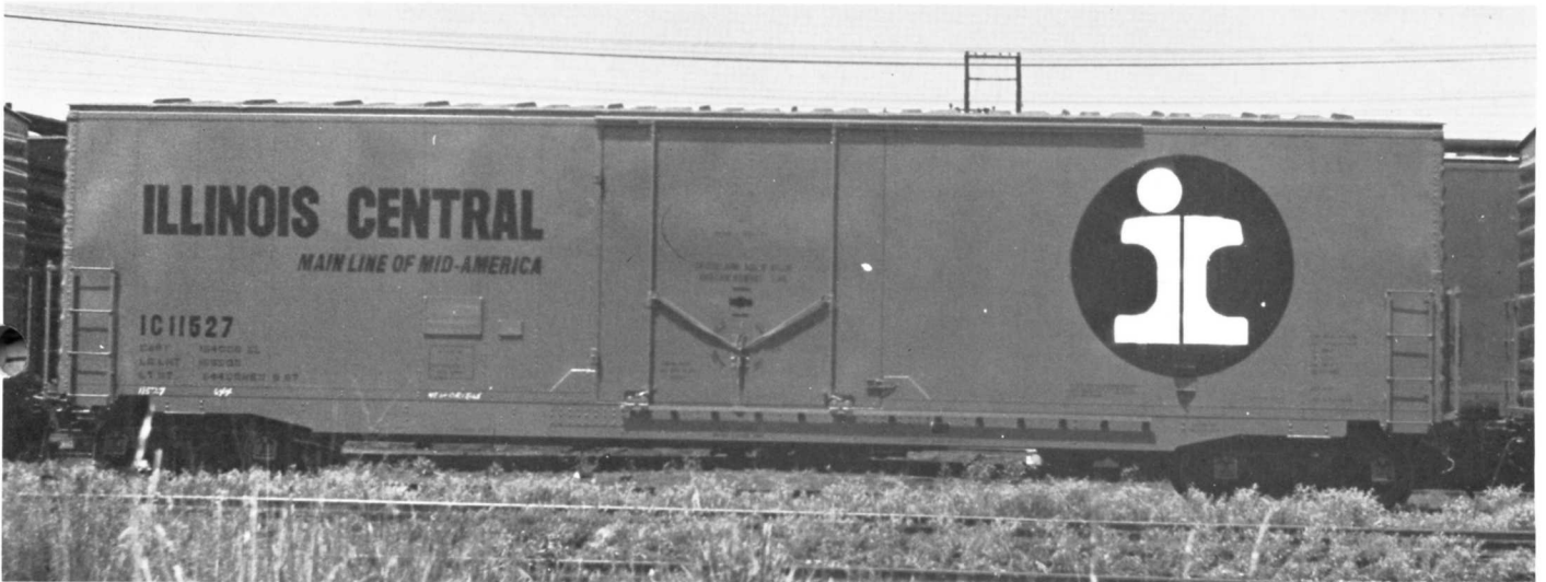
IC 11527 BOXCAR 50FT. PHOTO IC CENTRALIA SHOP EMPLOYEES - ICHS COLLECTION. 11500 to 11799 series built by the IC Centralia, IL car shop in 1967. Cars are equipped with DF-2 load devices.
